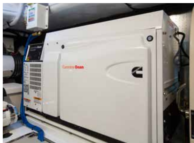
Double soft-mounted generator with proprietary hush chamber exhaust
