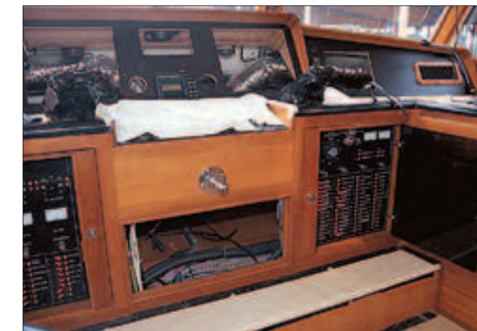
Careful preparation and effort results in holes measured twice, but cut once (above). The result—the completed pilothouse is both beautiful and functional (left).
